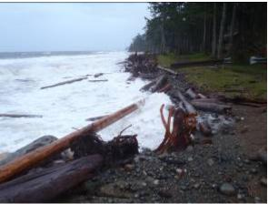
Shoreline protection at Kitty Coleman Provincial Park using ballasted trees before treatment (top left), during installation (top right) and after installation (above). During Nov 24, 2011 storm (above right) and day after (right).
