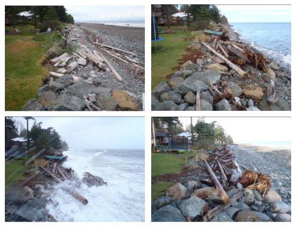
Shoreline armouring using conventional rip rap showing effects to neighboring property (top left) and restoration after using rooted tree revetment (top right). During Nov 24, 2011 storm (bottom left) and day after (bottom right).
