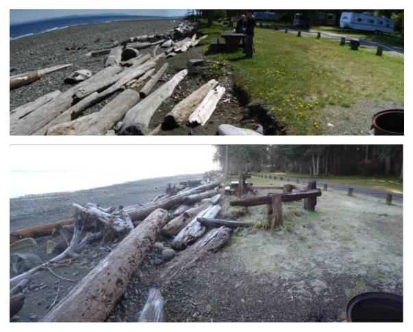
Shoreline protection at Kitty Coleman Provincial Park using ballasted trees before treatment (top) and 2 years after installation (bottom). Since treatment this segment of shoreline has been exposed to 2 storm events on Jan 18, 2010 and Nov 24, 2011, both estimated to have a magnitude 5 year return period.
